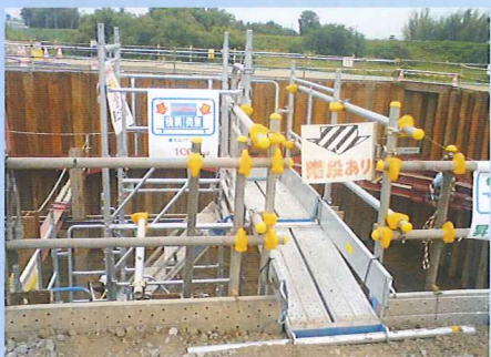
↑ 昇降口の施工例①
